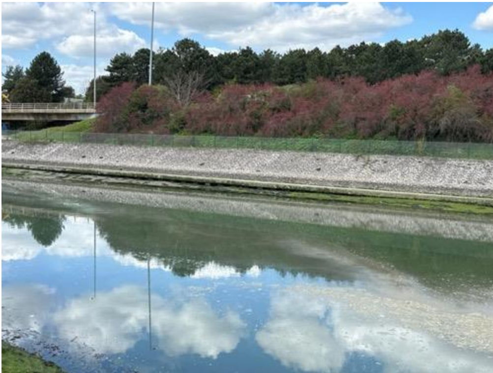
Photograph Z.8.4. Hard Engineered Edge Protection
