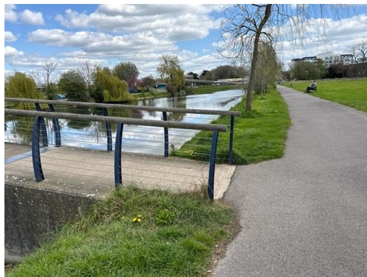
Photograph 2 : Bridge Across Waterbody
