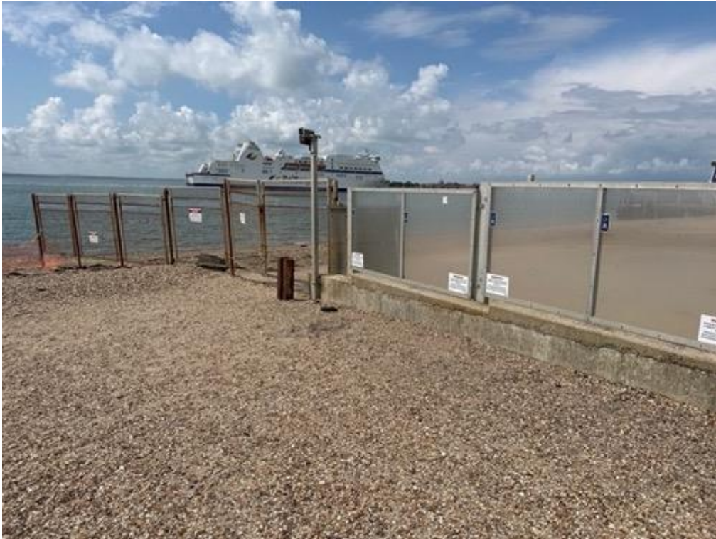
Photograph Z.2.a.1: Hoverport with Edge Protection and Warning Signs
