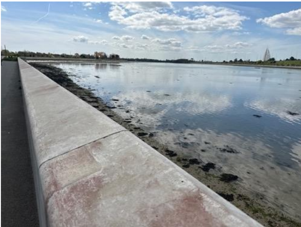
Photograph Z.8.3. Hard Engineered Edge Protection
